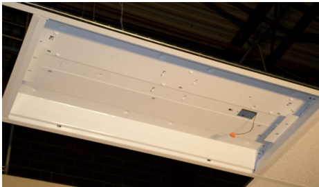
2) Insert endcaps between ceiling grid and troffer.
